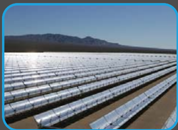
Nevada Solar One
